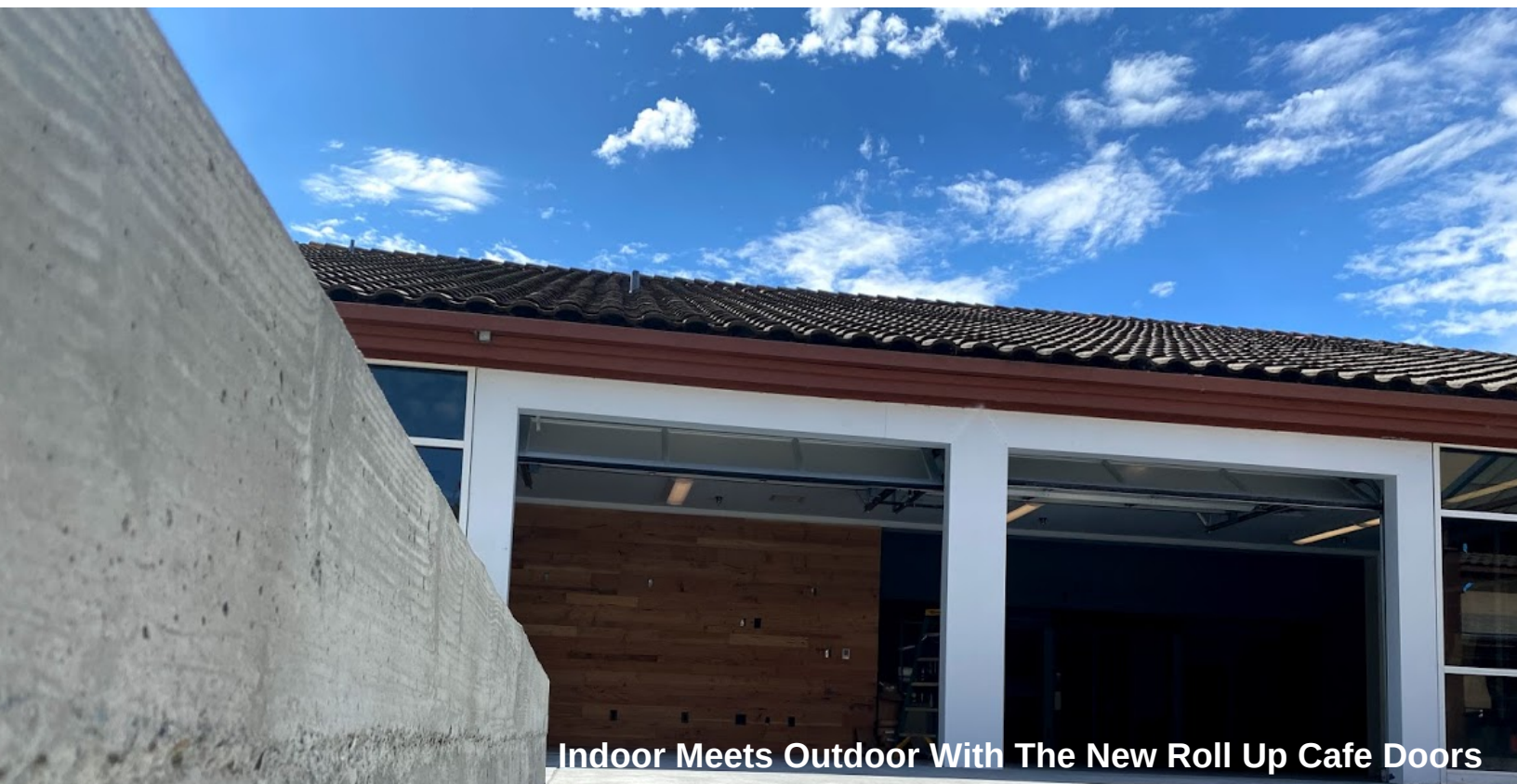
The Courtyard Cafe Concrete Pour Shapes the Space
